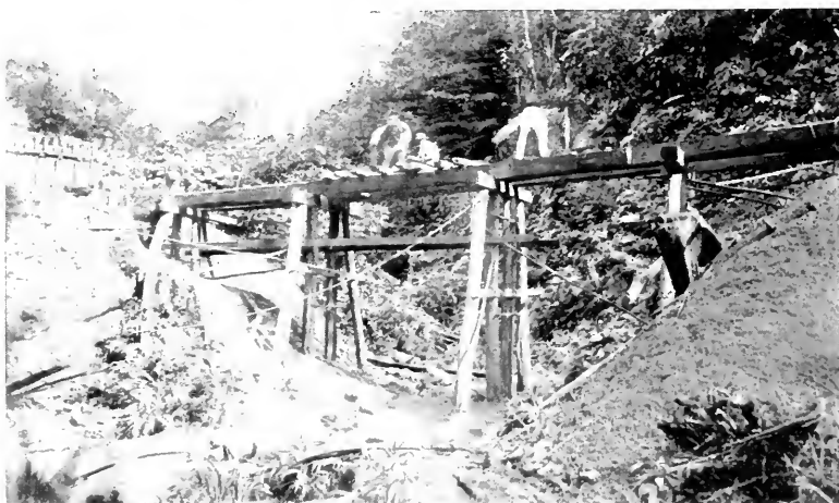
CONSTRUCTION OF BRIDGE NO. 38.
